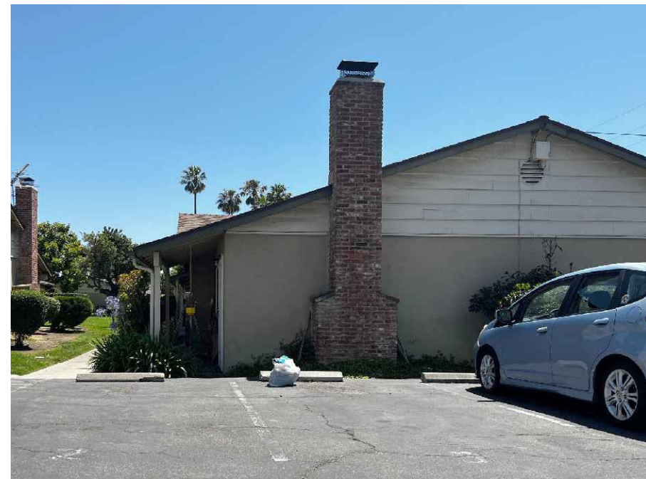
VIEW OF ADJACENT MULTI-FAMILY DWELLING
