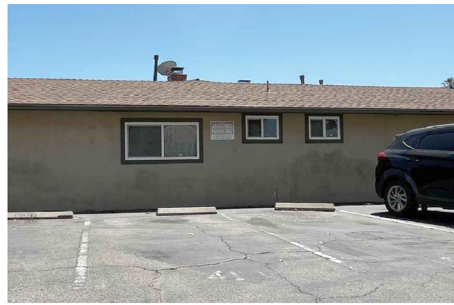
VIEW OF ADJACENT MULTI-FAMILY DWELLING
