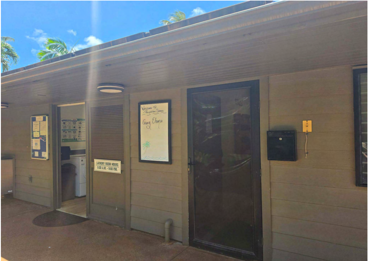
On-site facilities serving guests.
