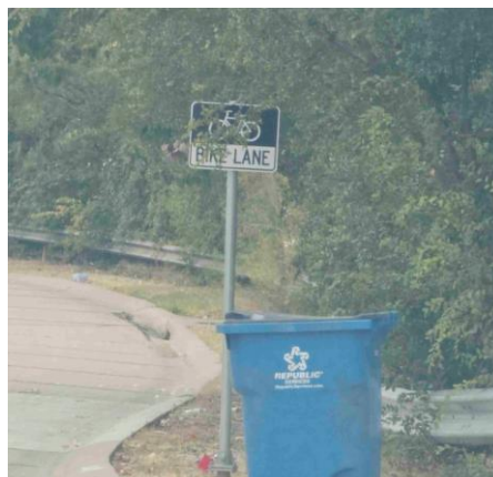
The Bike Lane sign at this transition can be partly obscured by foliage. Pavement-level guidance would provide an additional safety cue that does not depend on a single sign.
