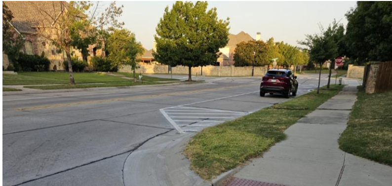
Nearby Lady of the Lake example showing advance pavement guidance. Pavement markings before bump-outs should provide consistency to help drivers stay in the intended driving lane and slow travel speeds.
